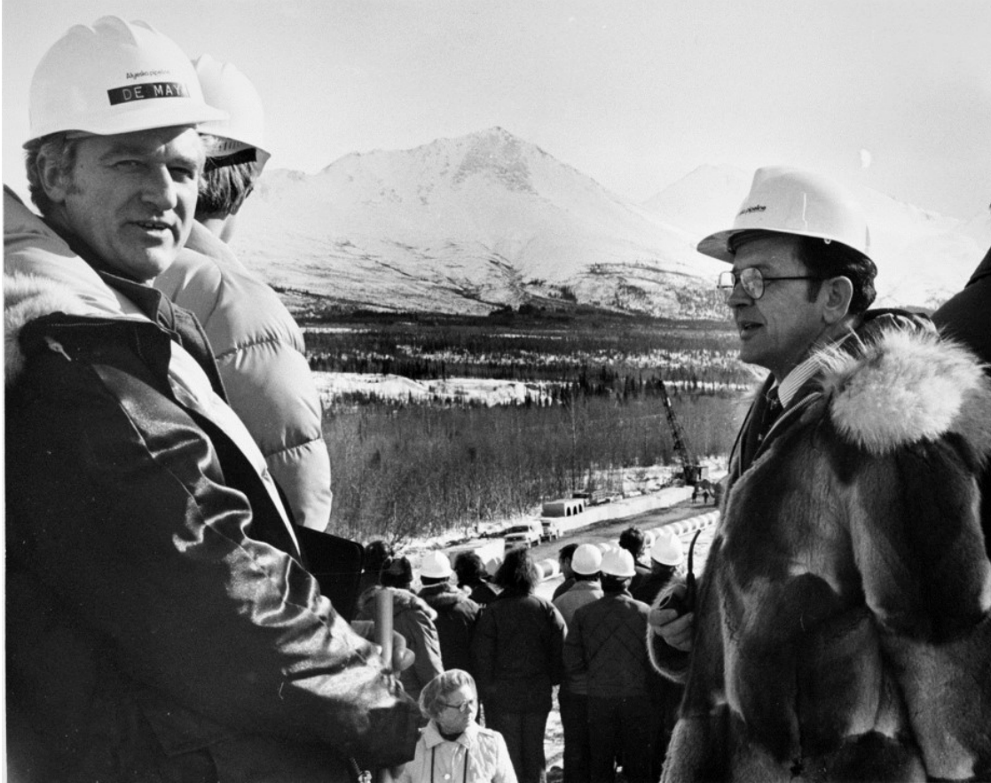
(Above) Senator Stevens, right, at Trans-Alaska Pipeline Tonsina River crossing, on the first day of laying pipe on March 27, 1975. Mike Dalton / Stevens Foundation photo.
